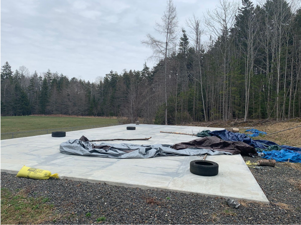
Construction of the St. George Makerspace Building has begun.
